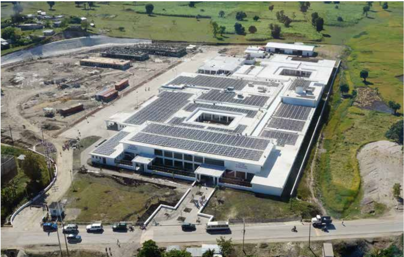
An aerial view of University Hospital of Mirebalais, Haiti, reveals 1,800 solar panels on the hospital's rooftop. The 205,000-square foot, 300-bed facility provides primary care services to 185,000 people in Haiti's Central Plateau, as well as secondary and tertiary care to all of central Haiti and the city of Port-au-Prince. (Photo: Rebecca E. Rollins / Partners In Health)
